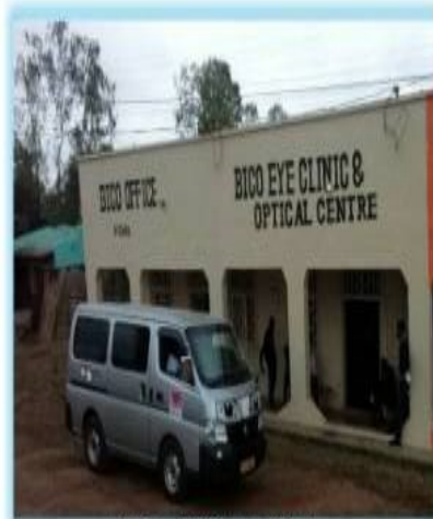
Ntcheu BICO eye Clinic along M1 Road Near Engen Filling Station
